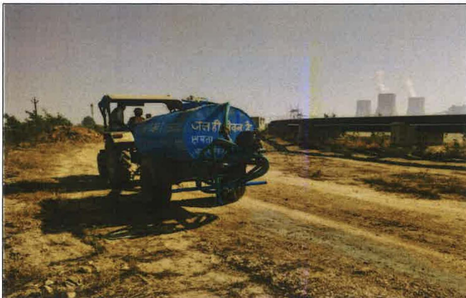
Fig 8: Water Sprinkling at Ash pond bund
