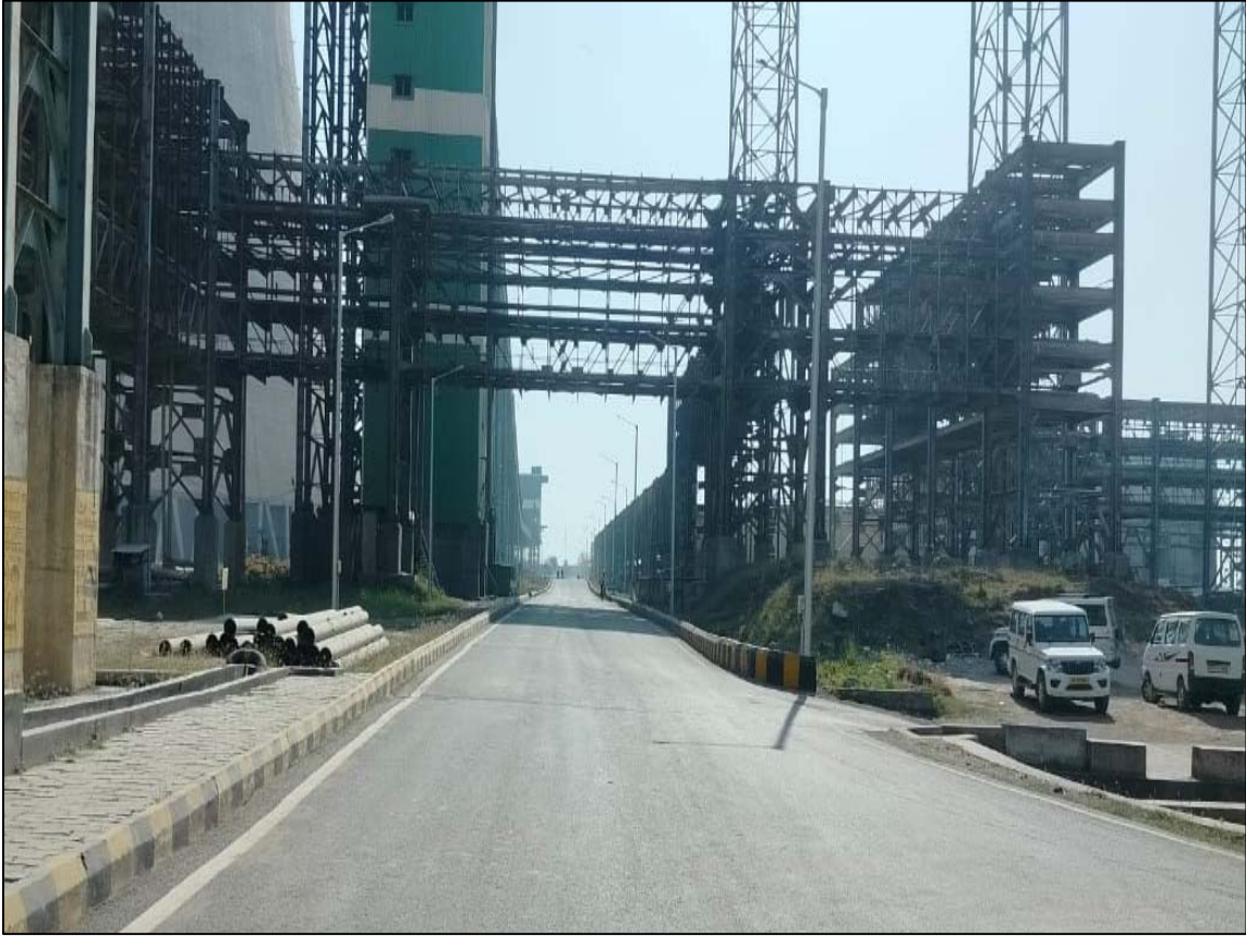
Service Building to JNT-2
