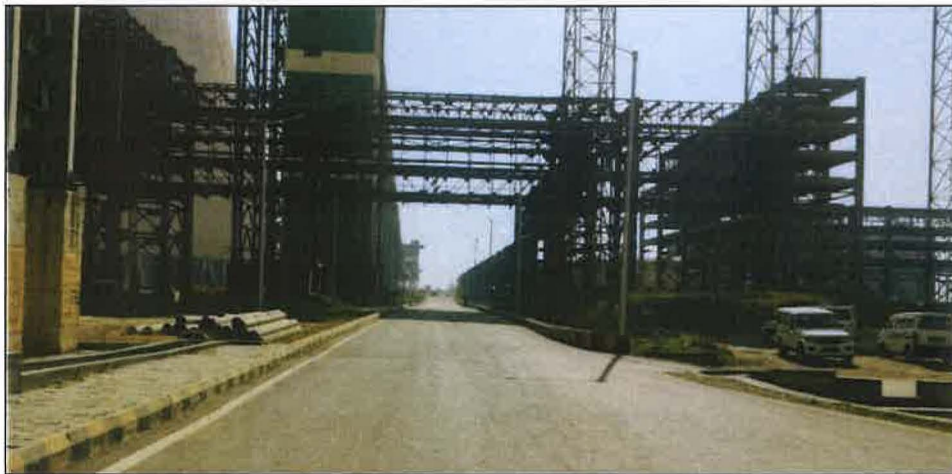
Fig 7: Service Building to JNT-2
