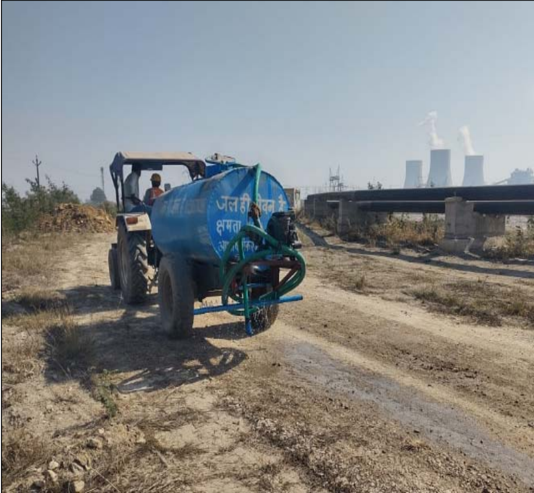
Water Sprinkling at Ash pond bund
